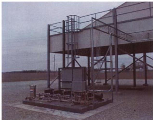
Fig. 1 Typical gas turbine inlet fogging skid
